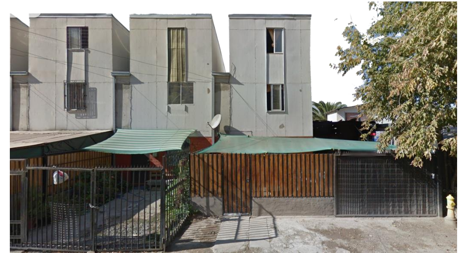
Stage I. Incremental housing complex – Image from 2012 – Google earth
