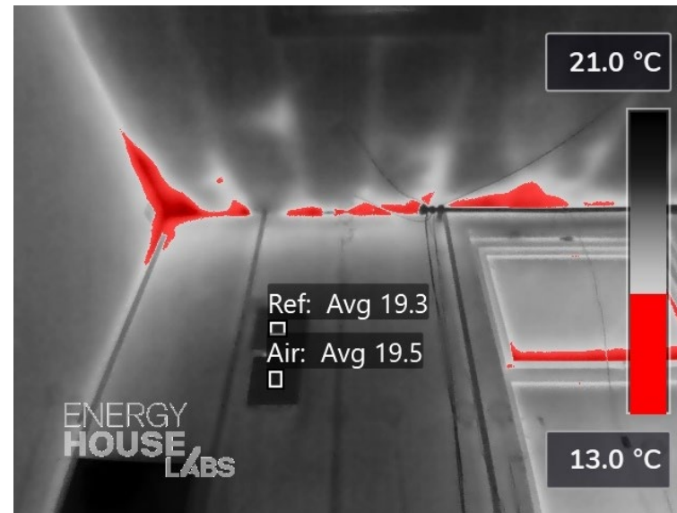
Stage 5 – EWI retrofit
