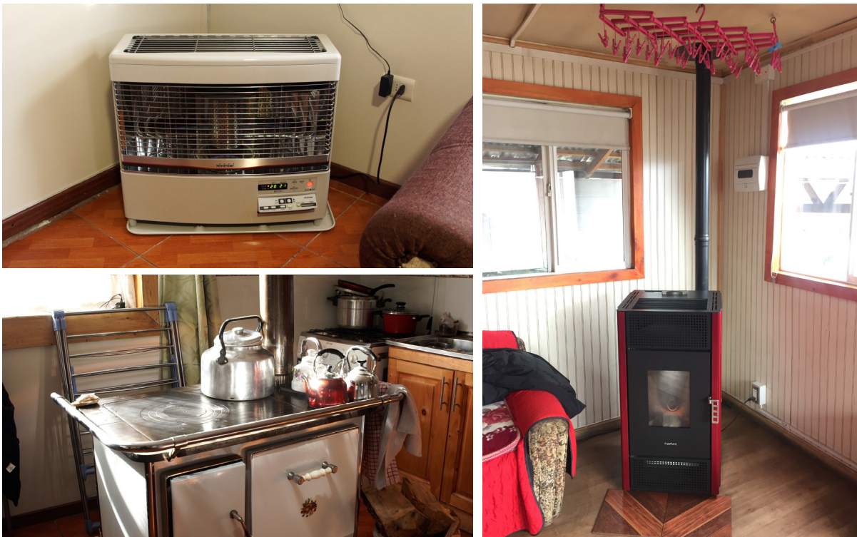
Clockwise from top left: Figure 4: Kerosene Heater Installed with the ADP Programmes Figure 5: Pellet Heater Installed with the ADP Programmes Figure 6: Woodstove in Coyhaique city Source: Authors, August 2022
