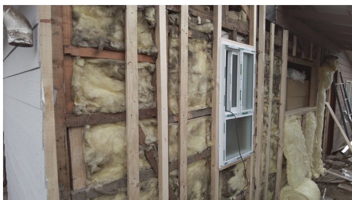
Figure 7: Wall Insulation Installed with the ADP Programmes. Source: Authors, August 2022
